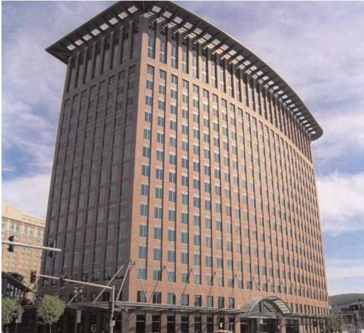
World Trade West Office Building Boston, MA
